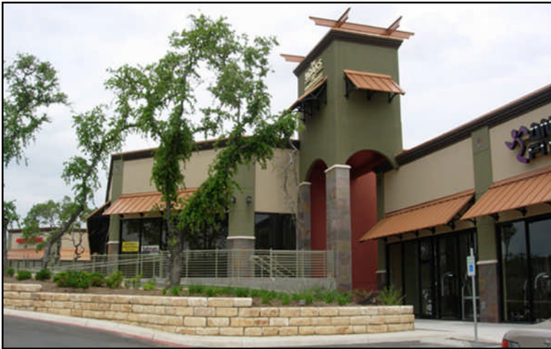
The Oaks at Green Valley Schertz, Tx
