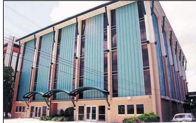
North Crown Office Building Renovation San Antonio, Tx
