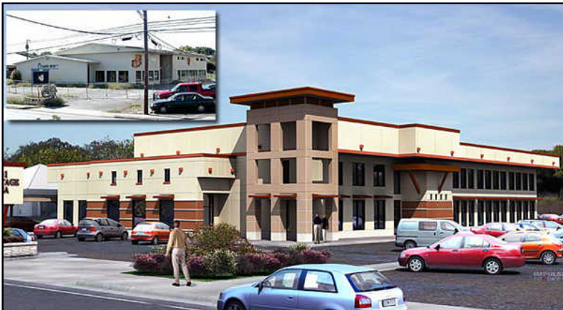
Advantage Plaza - 2 Story Office Renovation San Antonio, Tx
